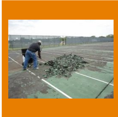
Outdoor Tennis Court Flooring Service
